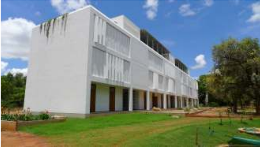
East facade of Luminosity
