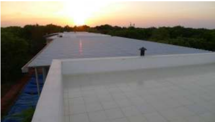
Roof of the head-rooms
