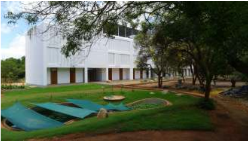
Polishing pond, part of grey-water-system
